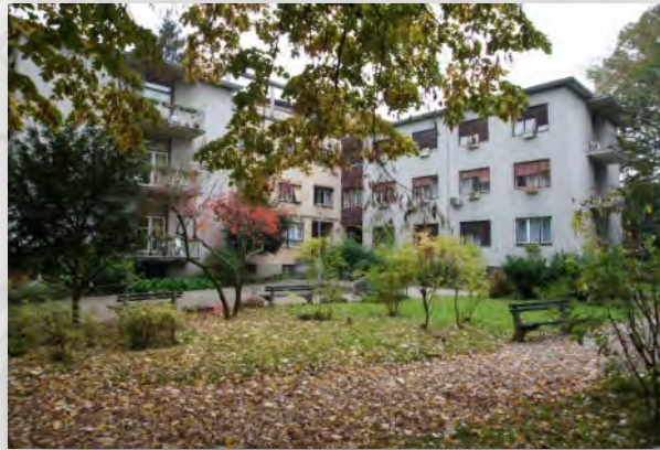
The new home for elderly people of the Lavoslav Š Schwarz Institute in Bukovačka.
