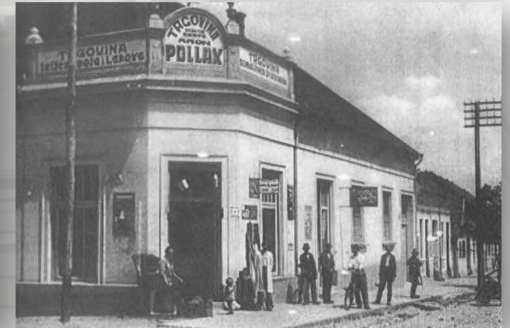
Paint and varnish shop in Našice
